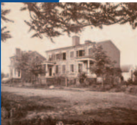
Battle-damaged homes in Fredericksburg
